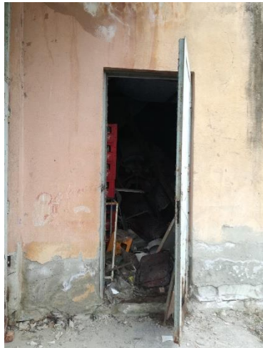
Pereti degradari – punct termic
